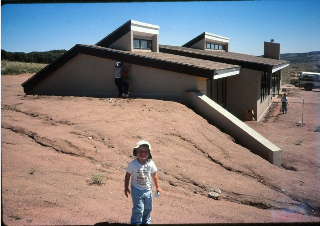
Beasant Residence (2500 sq.ft.) Construction progress photos: semi earth-sheltered, passive solar home in Sedalia, Colorado. Design and CM services by RBA, 1985.
