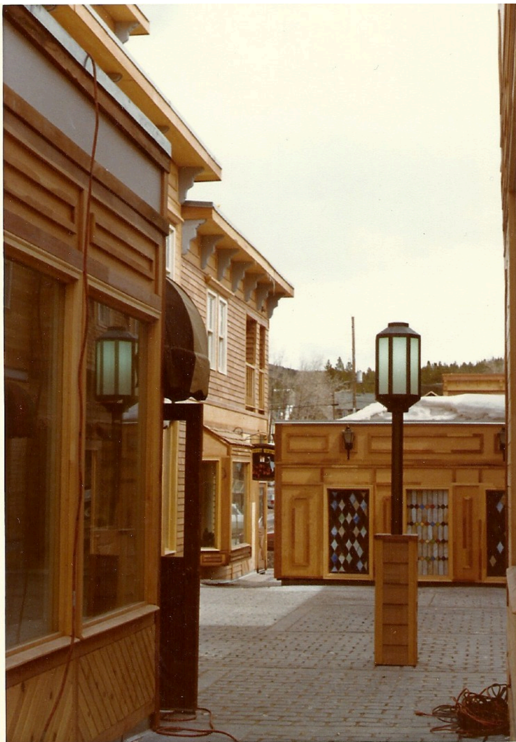
Construction progress photos of Georgian Square prior to completion in December, 1978 .
